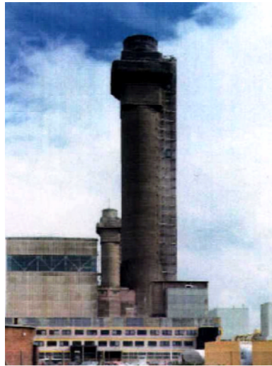
Figure 13: Windscale Pile Chimneys
