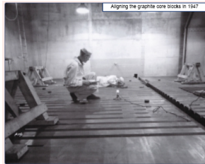
Figure 2: View of the GLEEP moderator under construction at Harwell
