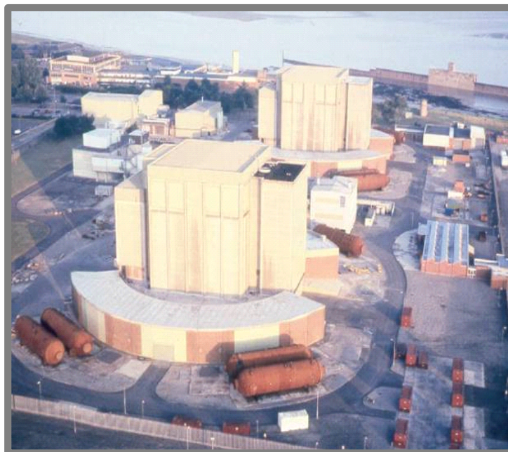
Figure 14: Berkeley Reactor Buildings
