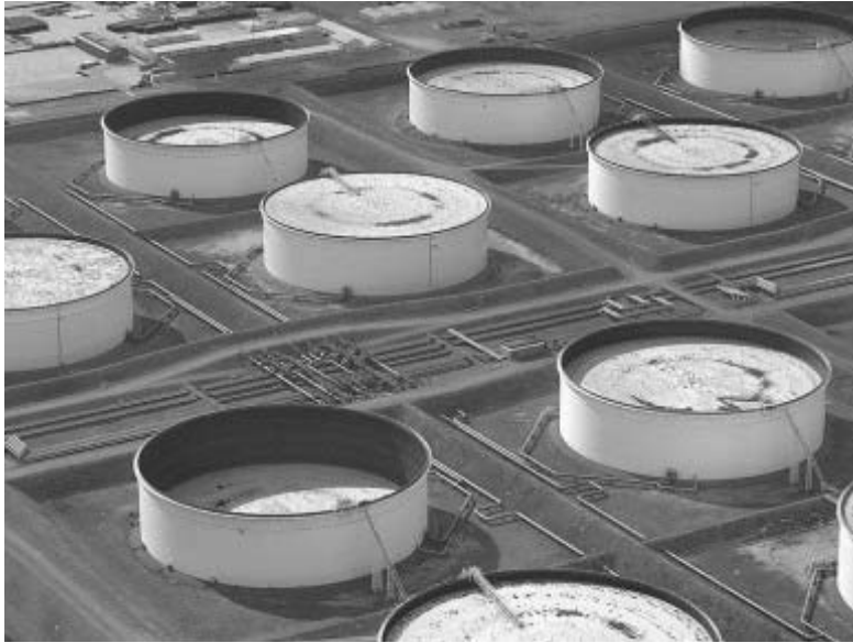
Figure 3-1 : Aerial view of crude oil storage tanks
