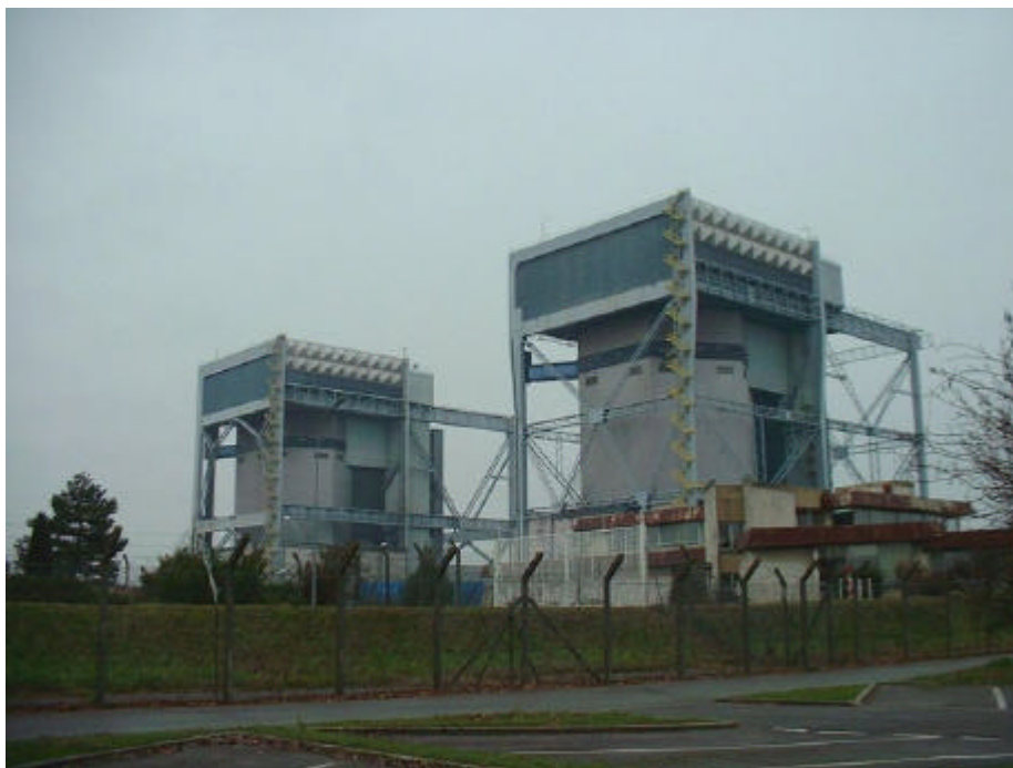
Figure 3.12 Saint-Laurent A1 (left) and Saint-Laurent A2 (right) UNGG reactors (current state 2012)
