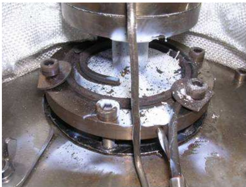
Figure 6. Union between chlorinator outlet and injection pipe inlet.
