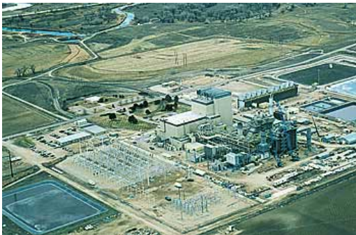
Fort Saint-Vrain, US (300 MWe, operated 1976-89)
