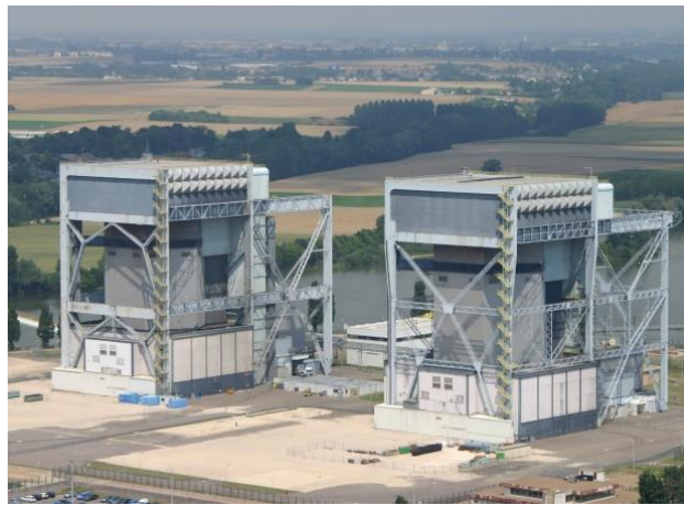
Figure 3.3.2: Saint-Laurent A1 (left) and Saint-Laurent A2 (right) UNGG reactors (current state 2012)
