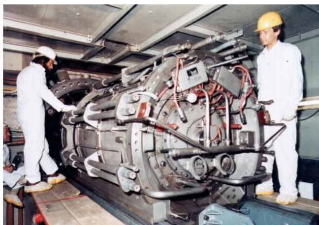
Figure 3-4: Installation of a THR-300 helium blower.
