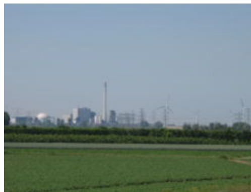
Figure 5: Borssele Nuclear Power Plant 10
