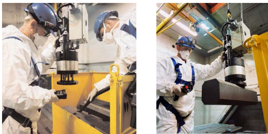
Figure 16 Sampling and Retrieval operations at GLEEP
