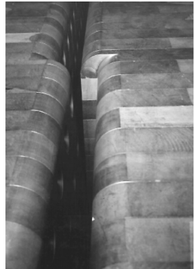
Figure 1 : Brookhaven Graphite Research Reactor, cut-out section through core and view of graphite blocks (from Brookhaven Graphite Research Reactor (BGRR) Decommissioning Project presentation by T Kneitel, October 2007).
