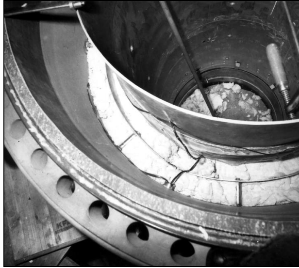
Figure 81: Mounting state (fibre insulation)
