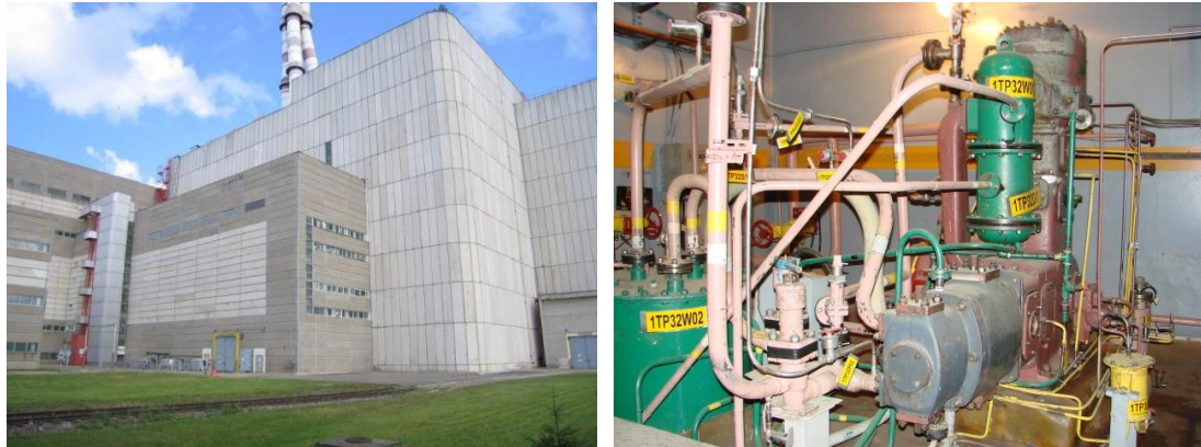
Figure 1: Building V1 outside and inside view
