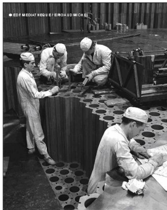
Figure 8 : Stack of graphite columns during Chinon A3 building in 1965
