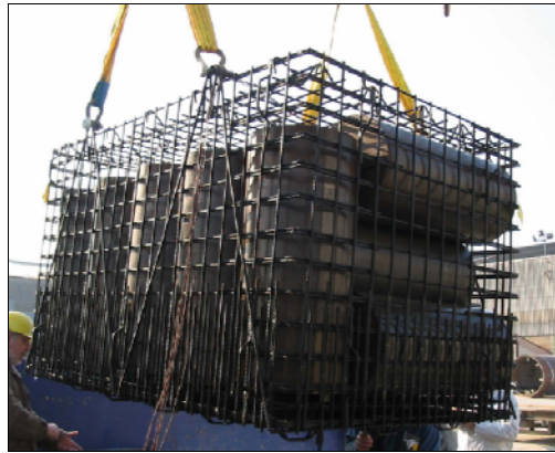
Figure 21 : Metallic basket with graphite (non irradiated for development tests here) to be grouted inside the concrete package.
